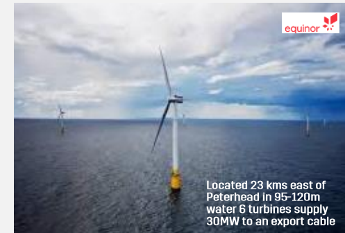
Hywind Scotland floating wind farm
